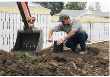
When required the FTB30 can be installed under the 8" and 10/12" Footing Tube (adds 90% more load bearing area)
